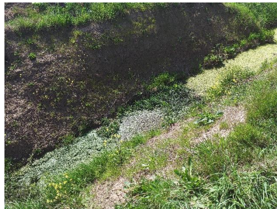
4: NVC ditch surveys – quadrat 7.1. Mown banks, recent dredging, ditch dominated by Callitriche stagnalis agg.
